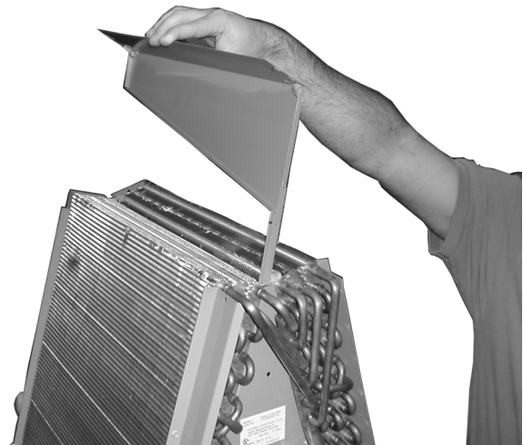
FIGURE 9 ROTATE DRAIN TROUGH
