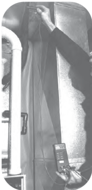
FIGURE 43 TEMPERATURE RISE MEASUREMENT
