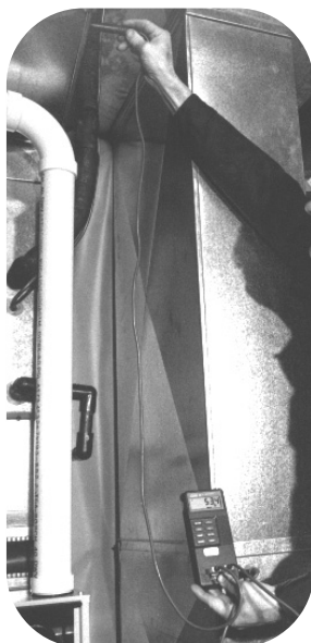
FIGURE 49 TEMPERATURE RISE MEASUREMENT
